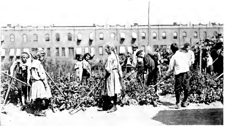
Fig. 150.—Crippled and defective children gardening (Playgrounds Association of Philadelphia).
