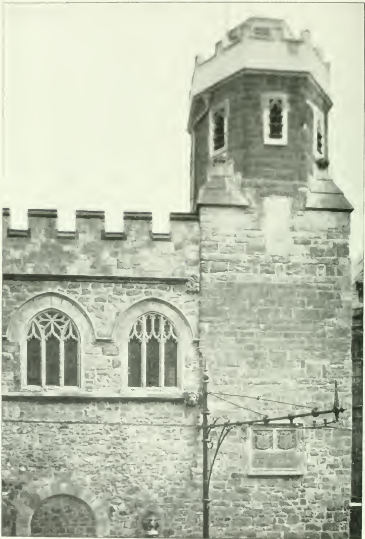
Tower of St. Petrock's.
