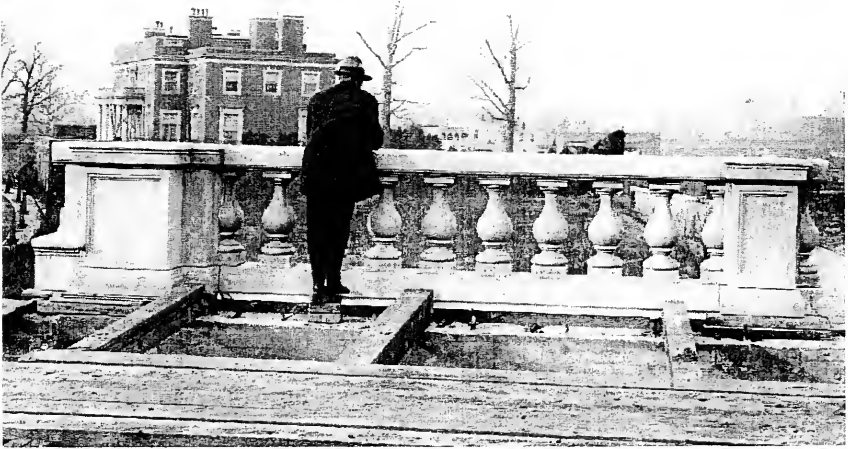
Figure 19: Baluster Mock-up, n.d (c. 1915-18) Rock Creek Park, Cultural Resource Management Archives
