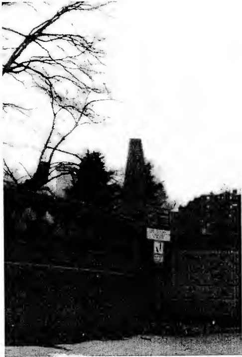
Figure 51: Missing Sphere from Obelisk at Southwest Entrance
