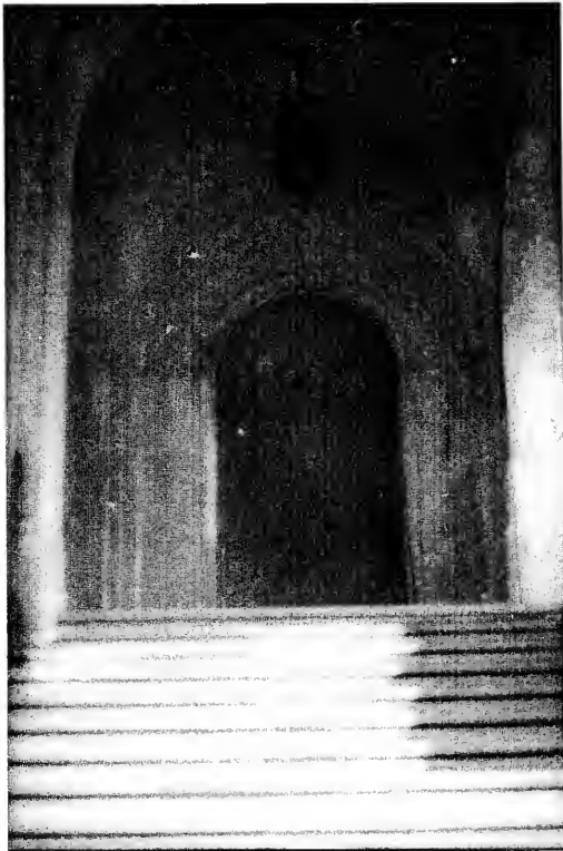
Figure 21: Interior of Main 16 th Street Entrance
