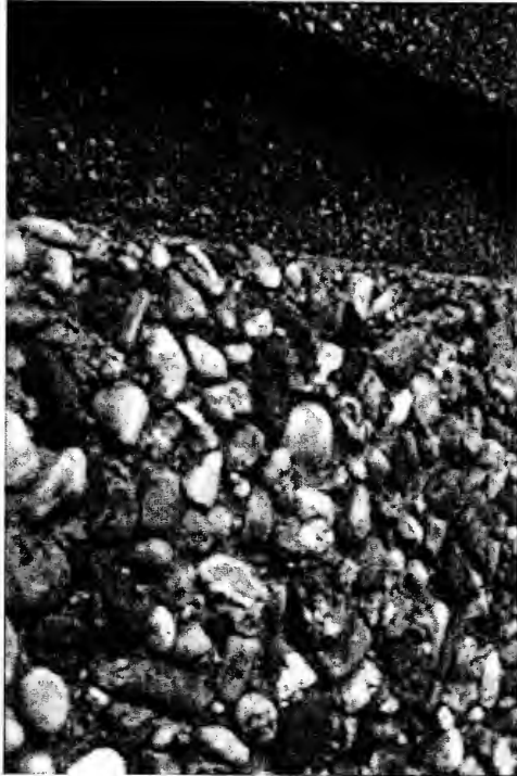
Figure 10: Detail of Coarse and Fine Textures, 1915 Construction
