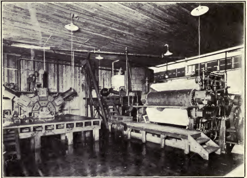
FIG. 2.—GRINDER AND WET-MACHINE ROOM.
