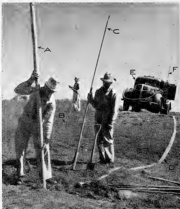
FIG. 539.—Approved procedure for loading shot holes. A, explosive; B, cap wires; C, loading poles; D, hose for filling hole with water; E, shooting truck with water tank; F, radio antenna. (Courtesy of Standard Oil of New Jersey.)
