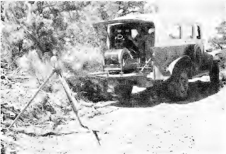
FIG. 617.—Radioactivity logging equipment for diamond drill holes: (A) cable; (B) tripod support for guide sheave; (C) reel; (D) recording equipment; (E) sheave wheel; (F) tripod brace.
