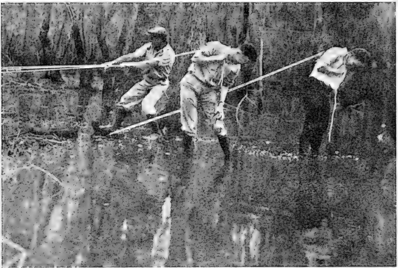
FIG. 531.—Laying cables in swamp areas.
