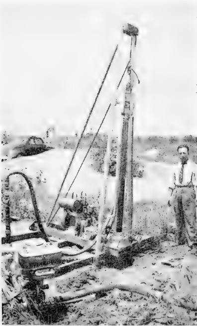
FIG. 554.—Light-weight seismograph drill. (Courtesy of Geophysical Service, Inc.)
