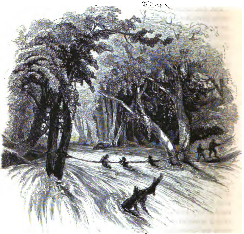
RUDE BRIDGE OVER THE OVIGUI.
