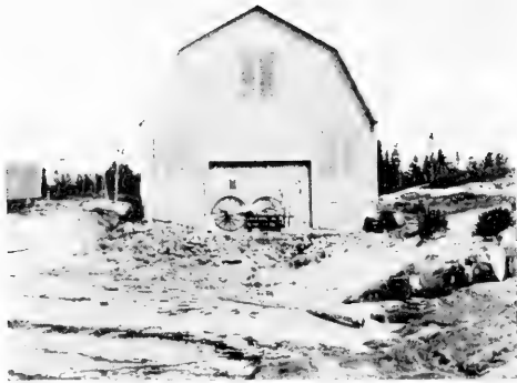
FIG. 78.—The “factory” on Mr. Copley Amory’s estate on Matamek River. This building functions as a boat house below, while on the upper floor is the working laboratory and storage for boat-dredges and fishing gear.
