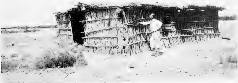
FIG. 164.—Pima houses are usually built of suhuaro cactus ribs, plastered with mud. When their water supply fails, the Pima move.
