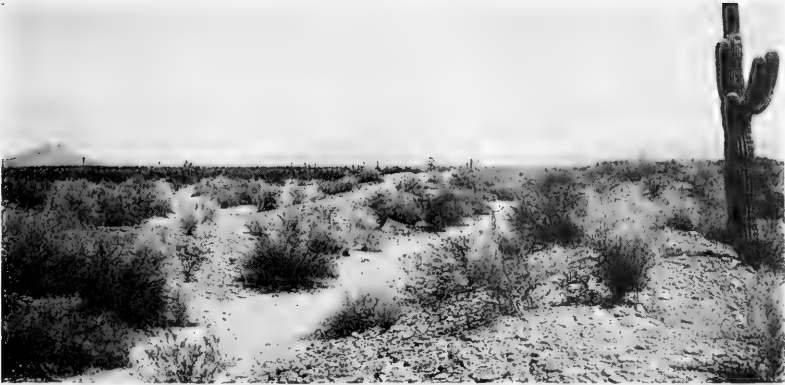
FIG. 162.—Near its present junction with Salt River, Canal Fourteen measures 8 feet deep with a maximum width of 66 feet.
