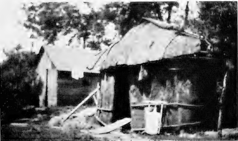
FIG. 208.—Fox building made of elm-bark, Tama, Iowa. (Photograph by Michelson.) Buildings of this kind are rapidly disappearing and will soon be a thing of the past. This building is one of the finest ever seen by Dr. Michelson.
