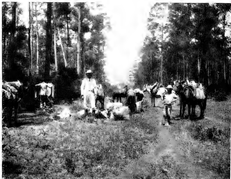
FIG. 40.—Adjusting pack panniers on the trail leading to Constanza. The sturdy mules carry heavy burdens without seeming difficulty. Taken May 29, 1927.
