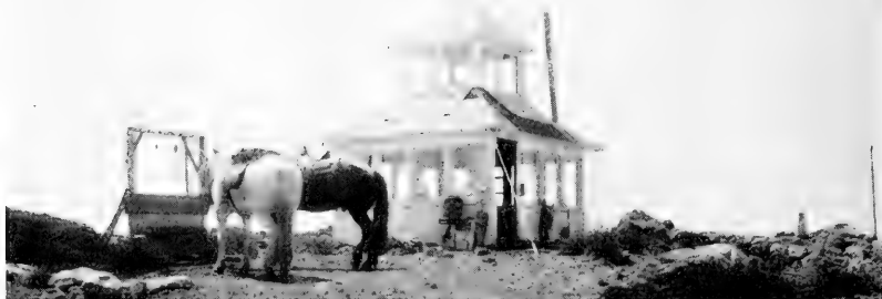
FIG. 117.—Lookout Station on Sanger Peak, northern California, in the Siskiyou National Forest. These stations are placed on the high peaks to aid in fire protection. A lookout man lives here during the summer months. He is on the watch for fires. The notice of a fire with its direction is at once telephoned to a central station. The living room is below, the observation room above.
