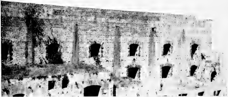
FIG. 51.—Section of wall of the famous Citadelle from the inside. The Citadelle was built by Cristophe, once emperor of northern Haiti, as a final stronghold against the French.
