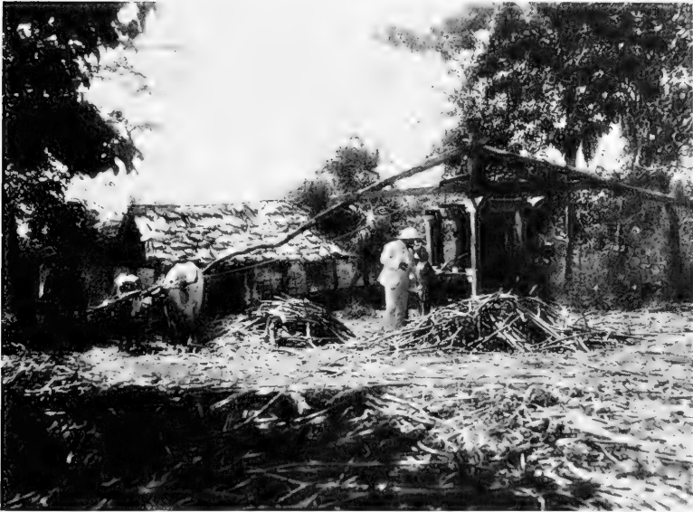
FIG. 35.—Native cane mill at the Artibonite River near Las Cahobes, Haiti, on the road to Hinche. The juice of the cane, expressed by heavy wooden rollers, is boiled over open fires in the shed in the background to make rapadou or crude sugar. Taken April 20, 1927.
