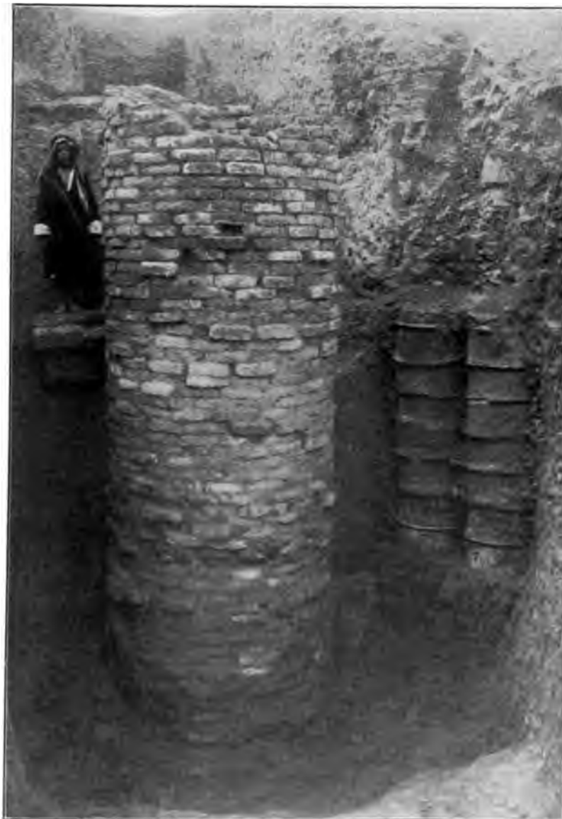
Well built of Bricks and Two Terra-Cotta Drains
