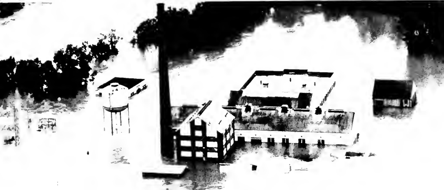
Tropical storm Albert dumped nearly two feet of rain, flooding the Flint and Ocmulgee rivers in the central and southwestern sections of Georgia.
