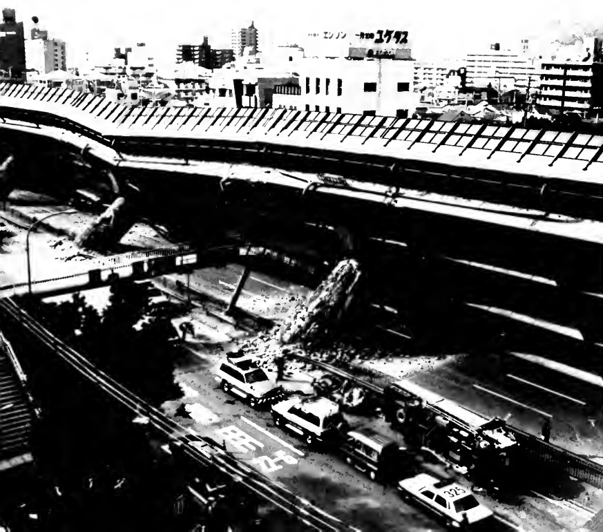
Japan's nightmare of a disastrous urban earthquake came true on January 17, 1995 when a powerful quake tore through several western cities, toppling hundreds of buildings.
