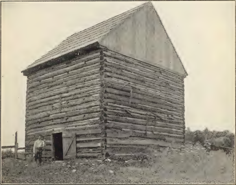
FIG. 13.—Common type of Virginia log barn for curing dark tobacco with open fires. (Photographed by the Bureau of Soils.)
