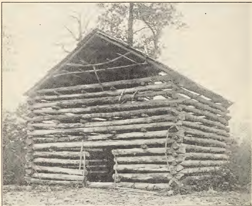
FIG. 9.—Early type of log curing barn for air-curing tobacco still seen in some of the Virginia, Kentucky, and Tennessee districts.
