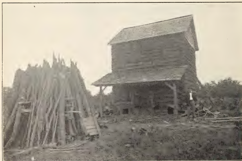
FIG. 24.—Typical flue-curing tobacco barn, Old Belt section, Pittsylvania County, Va. The pile of wood is for burning in the furnaces.
