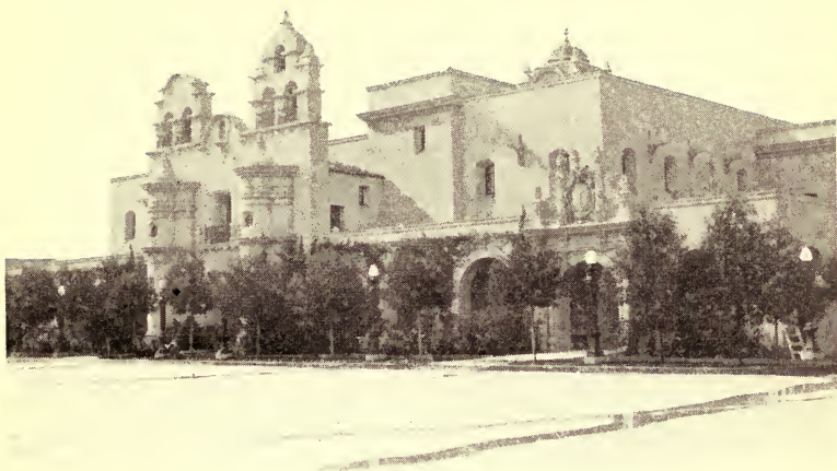
EAST FACADE, RUSSIA AND BRAZIL BUILDING
