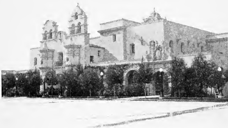
EAST FACADE, RUSSIA AND BRAZIL BUILDING
