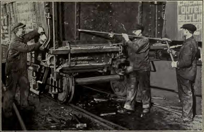
Fig. 16.—Cutting rivet heads.
