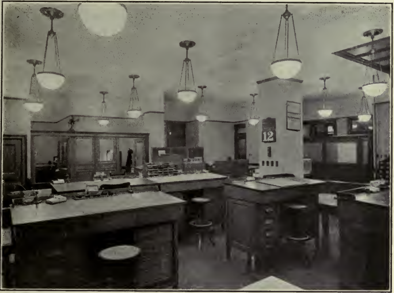
Fig. 46.—Semi-indirect office gas lighting. Note the absence of shadows even on the ceiling. Consolidated Gas Company of New York.
