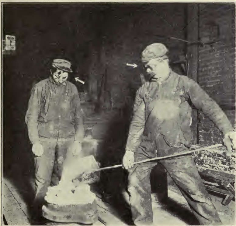
Fig. 20.—Pouring babbitt—single hand ladle. Carnegie Steel Company.
