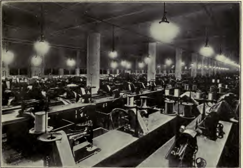
Fig. 41.—Lighting of sewing machines. Consolidated Gas Company of New York.
