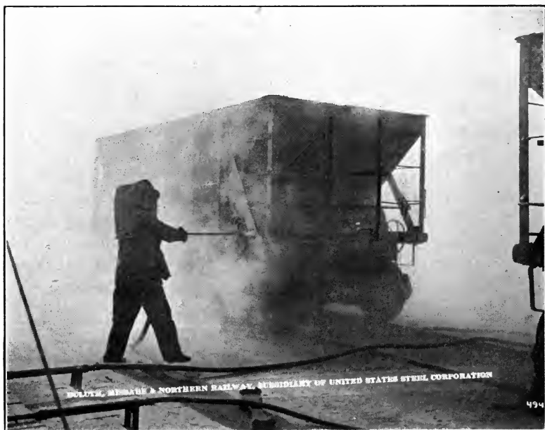
Fig. 11.—Hood used by men sand-blasting steel ore cars. Duluth, Missabe and Northern Railway.
