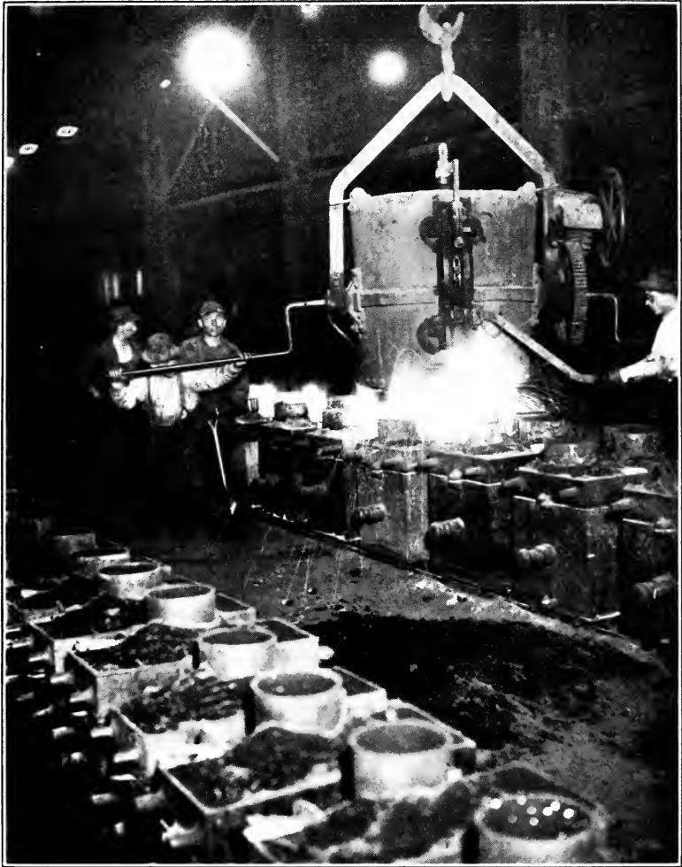
Fig. 21.—Pouring from bottom ladle. Only the operator is wearing protective goggles.
