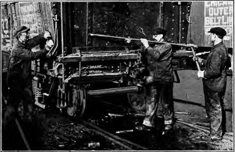
Fig. 16.—Cutting rivet heads.
