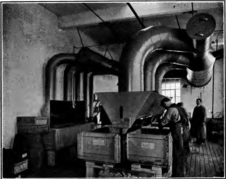
Fig. 33.—Ventilating System for Removing Acid Fumes. The suction opening is below the operator's breathing line, and no fumes reach his face. American Museum of Safety.
