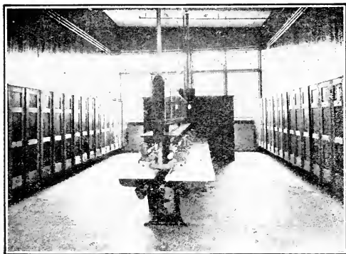
WASH ROOM AND LOCKERS (r)
