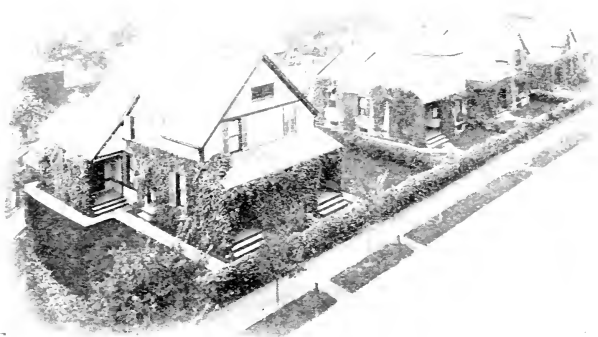
FRONT YARDS OF EMPLOYEES' HOUSES, DAYTON, OPPOSITE FACTORY (b)
