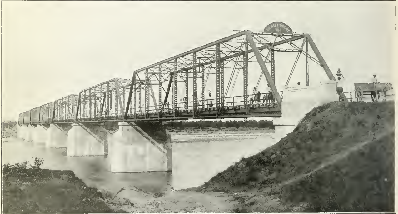
GILBERT BRIDGE, LAOAG, ILOCOS NORTE
