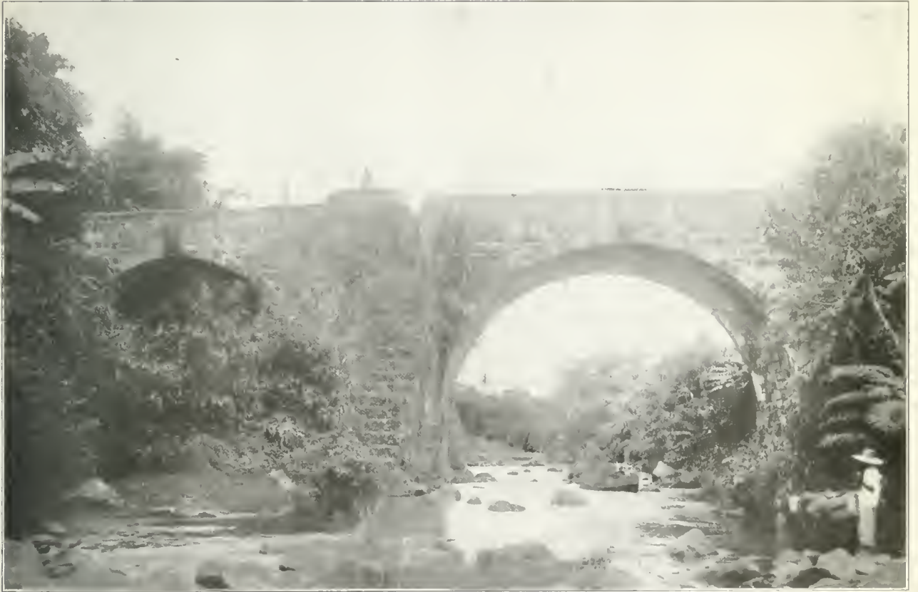
AN OLD MASONRY BRIDGE
