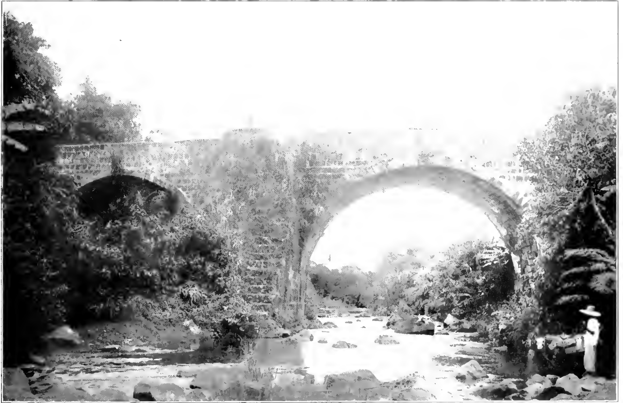
AN OLD MASONRY BRIDGE
