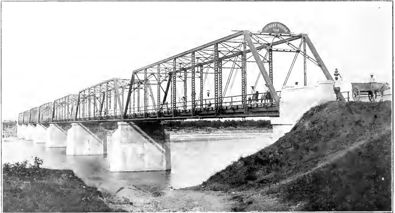
GILBERT BRIDGE, LAOAG, ILOCOS NORTE
