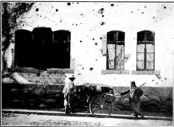
THE MOLTKE BARRACKS AFTER THE SURRENDER Showing the effects of Japanese shrapnel. Sandbags were placed about buildings in the city to keep shells from undermining them
