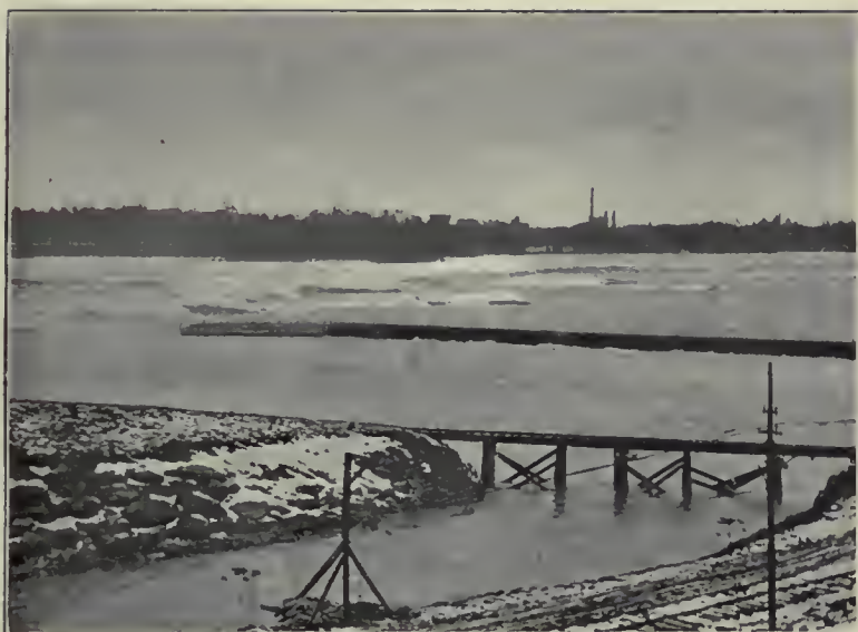
View of Greens or First Cascade across Ontario Power Co. Forebay, (from hill above western side of Upper Rapids).
