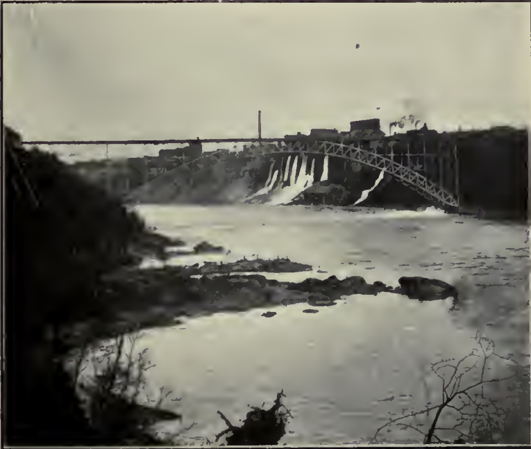
View of Carter Cove, Upper Arch Bridge, and factories on the N. Y. bank of the gorge beyond.
