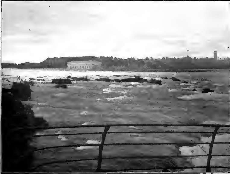
View of Goat Island shelf, adjacent to the Falls, which is being drained, with rocks appearing at surface. (Sept. 1906.) Electrical Development Company Power House in Victoria Park, shown in background.
