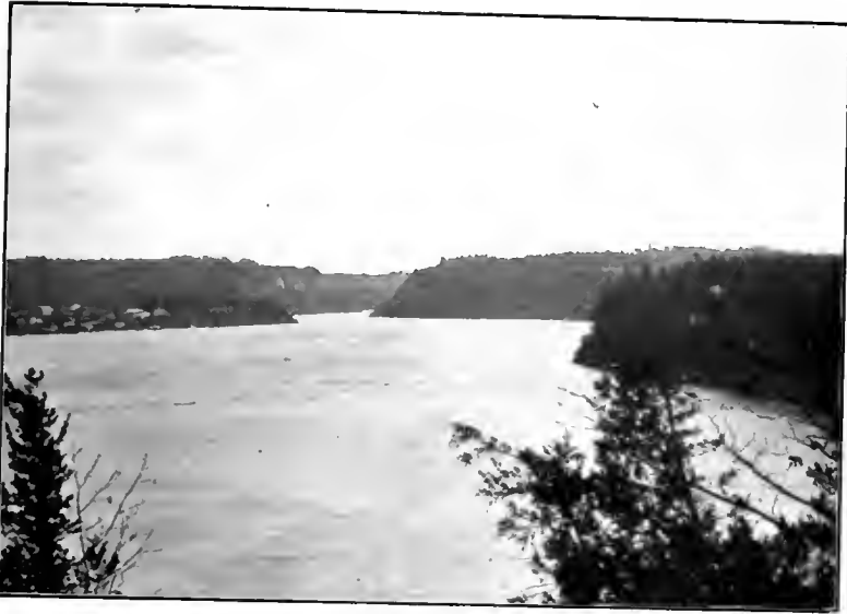
View of outlet of gorge cutting the Niagara escarpment (about 330 feet high with Brock's Monument, to the right).
