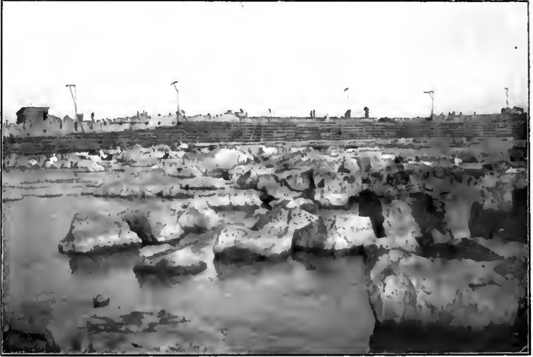
View of Bed of River at Electrical Development Company's Forebay when water was drained off. The joints in the bed rock opened by solution of the limestone, leaving separated masses still in place.
