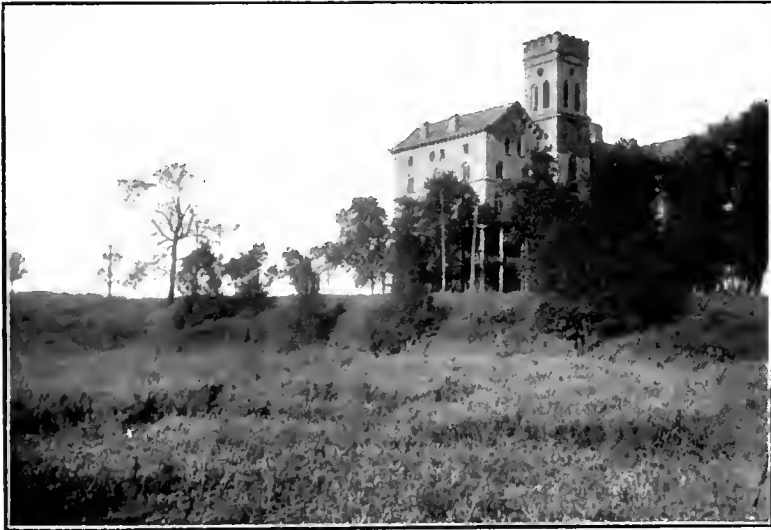
View of Original River bank, outside of the Narrows of Gorge, in front of Mount Eagle.
