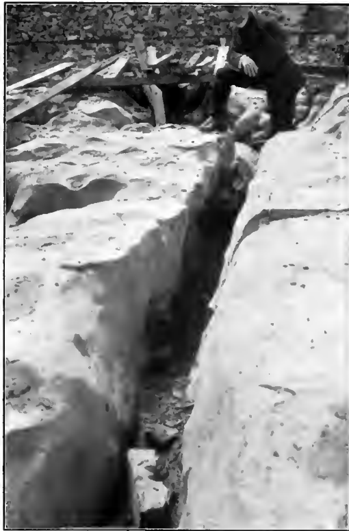
View of deep crevice opened in bedrock by the river currents at Electrical Development Company's Forebay.
