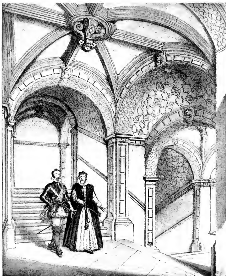
BURGHLEY HOUSE—THE STONE STAIRCASE.
