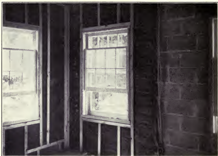
Figure 136. Furring strips separate plaster or other wall finish from the masonry wall. Blanket insulation placed between furring strips.
