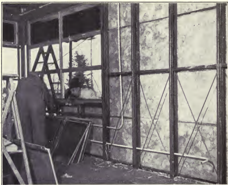
Figure 146. Erection of metal prefabricated frame. Note metal frame, tie rods, electric conduit, windows, and panels.
