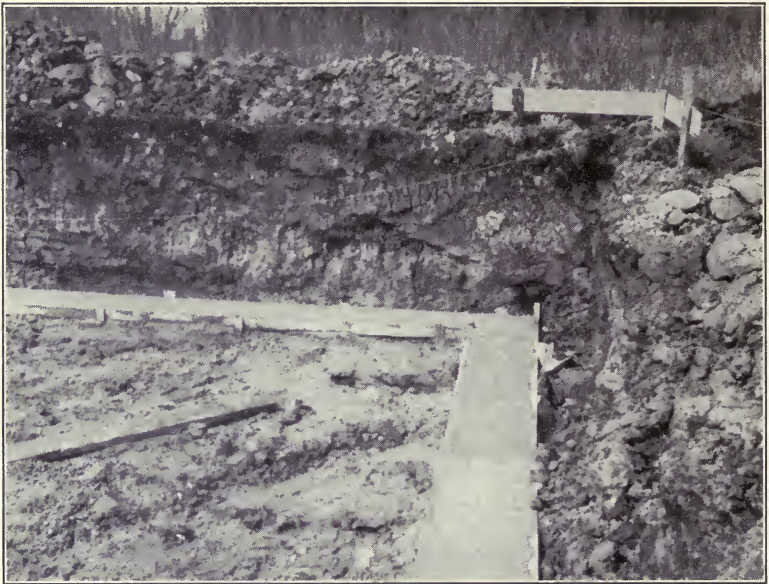
Figure 130. First steps in construction: Excavation and footings. Note "batter board" and chalkline.
