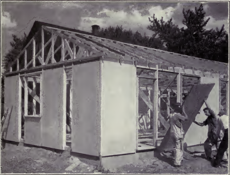
Figure 139. Applying manufactured panels on post and girder frame. See Figure 124.
