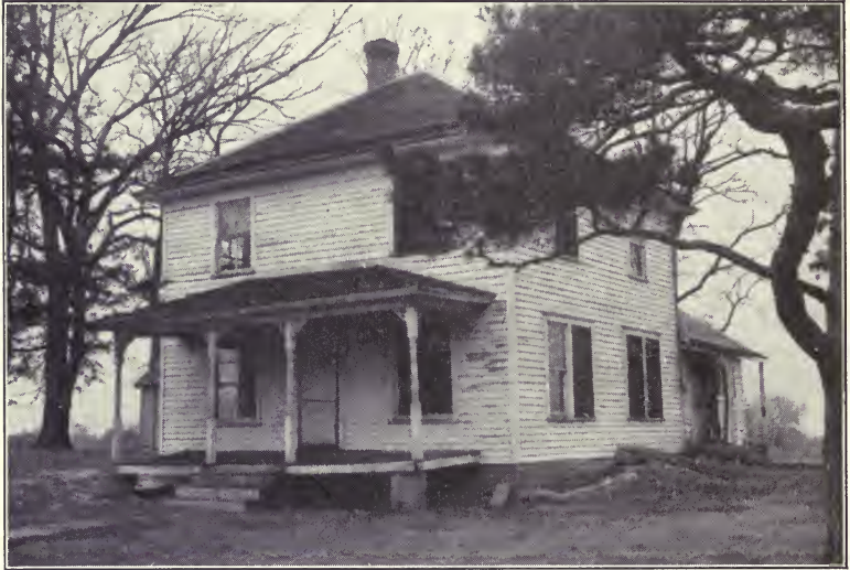
Figure 6. A typical example of the need for housing improvement. For one remodeling solution, see Figure 86.
