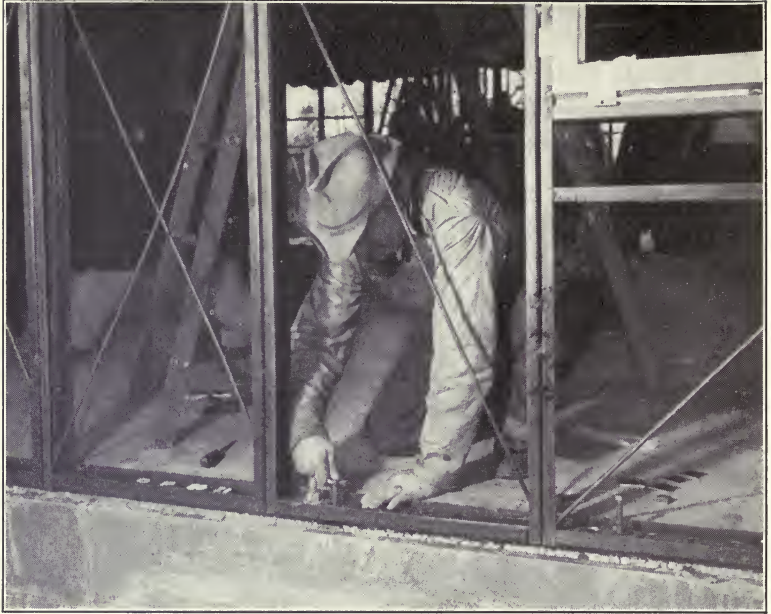
Figure 140. Use of metal in house framework.
