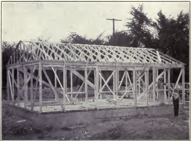
Figure 124. Modern adaptation of post and girder frame, used with wall panels.
