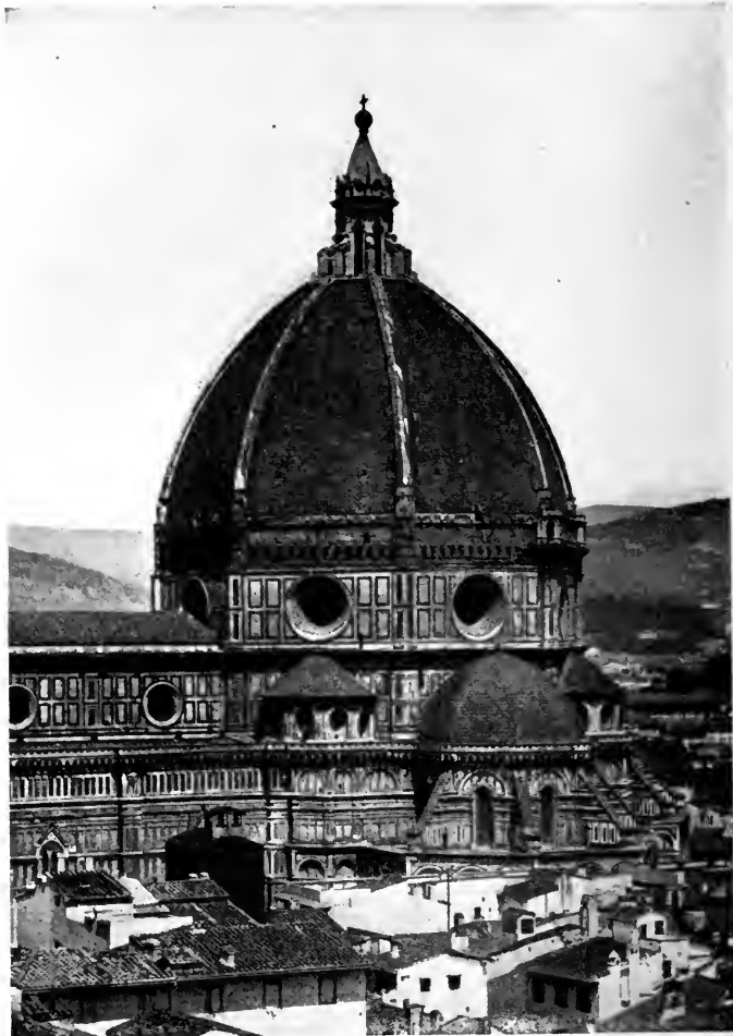
Fig. 72. The dome of the Cathedral, Florence, Italy. See description on pages 166 to 170.
