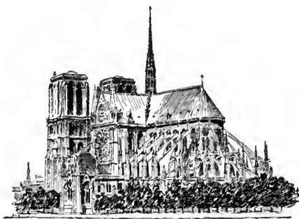
Fig. 61. View of Notre Dame Cathedral, Paris, from the southeast showing the great flying buttresses and the rood-steeple.
