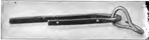
FIG. 49. SINGLE TREE HOOK AND STRAP.
