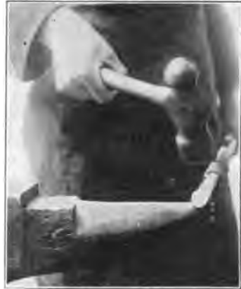
FIG. 43. BENDING POINT OF SCARF.
