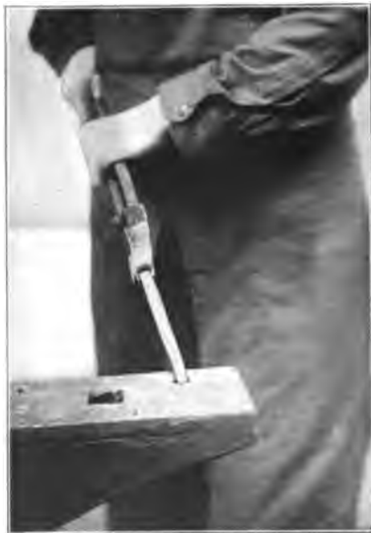
FIG. 21. BENDING IN THE PRITCHEL HOLE
