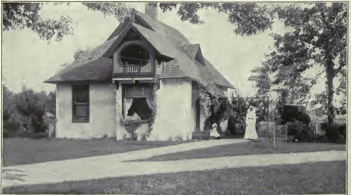
FIG. 399. OUTSIDE PLASTERING OF A FARM COTTAGE.
