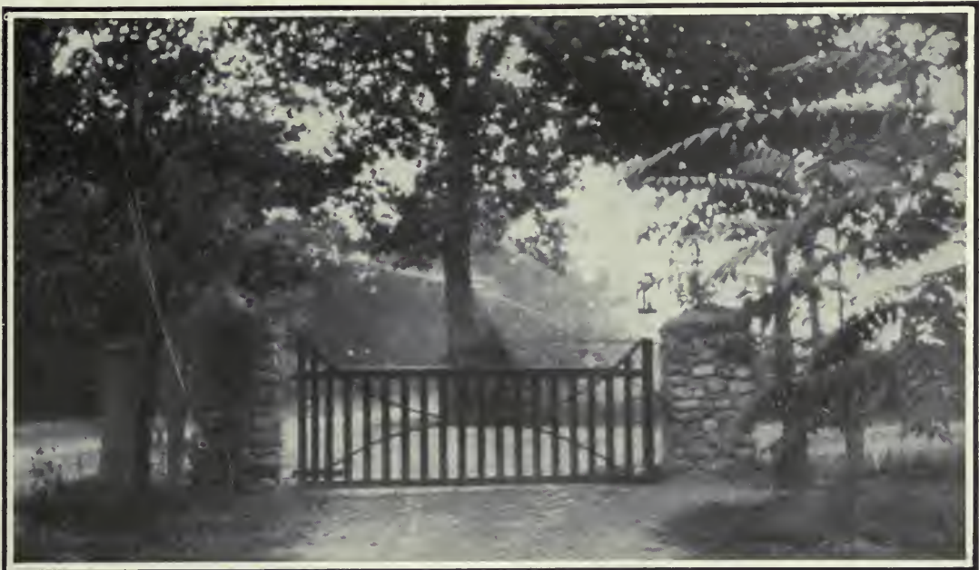
FIG. 388. CONCRETE RUBBLE WORK FOR GATE POSTS.
