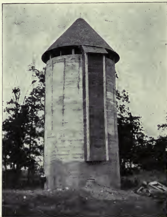
FIG. 403. WING CEMENT SILO.
