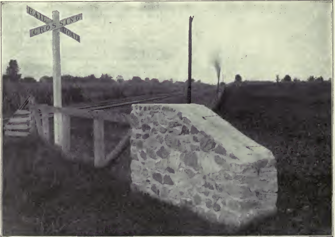
FIG. 480. STONE ANCHOR WALLS FOR FENCE.
