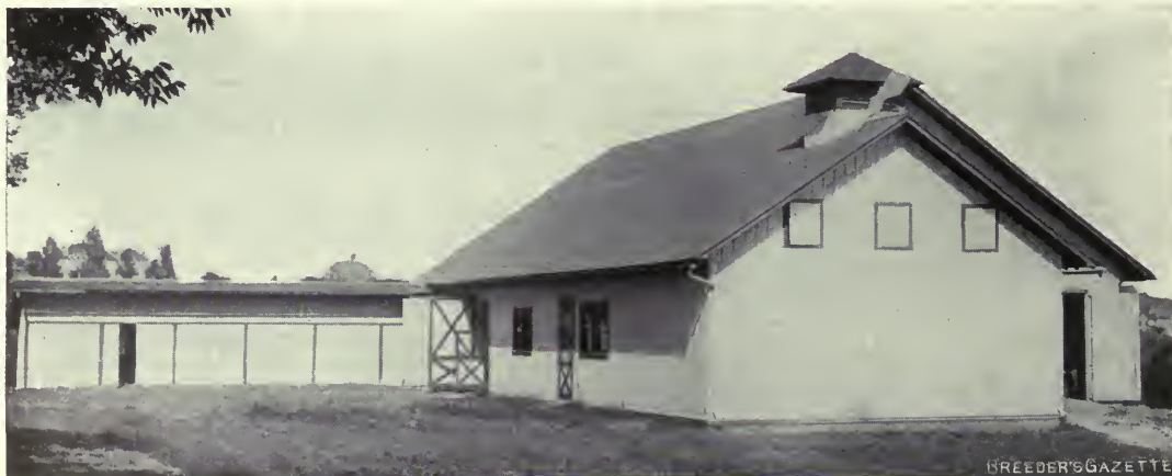
FIG. 246. TENNESSEE DAIRY BARN (SHED ADDITION).
