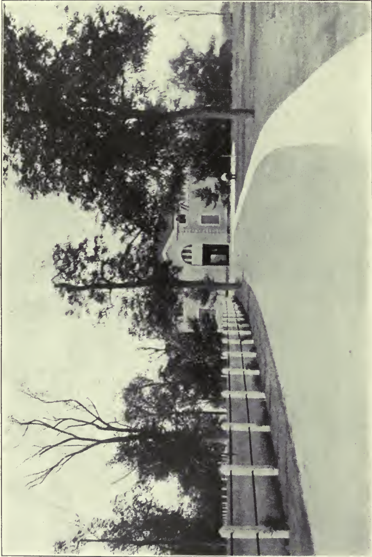
DRIVEWAY AND CARRIAGE HOUSE ON THE ELMENDORF FARM OF J. B. HAGGIN OF KENTUCKY. (Cement Fence Posts on the Left.)
