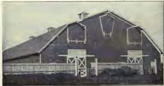
FIG. 182. A MULE BARN (REAR ELEVATION).
