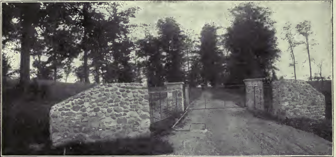
FIG. 479. STONE ANCHOR WALLS FOR FENCE.
