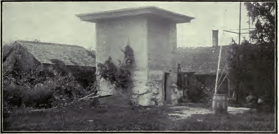
FIG. 394. CONCRETE WATER TANK.
