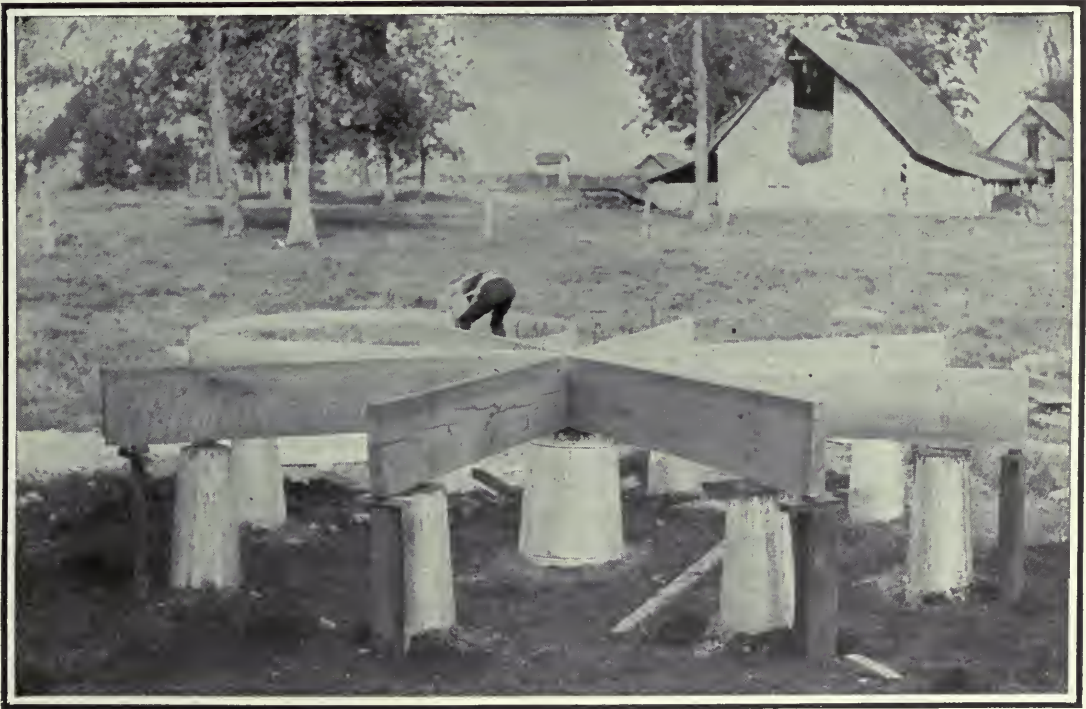
FIG. 421. ROUND RAT-PROOF CORNCRIB (CONSTRUCTION).
