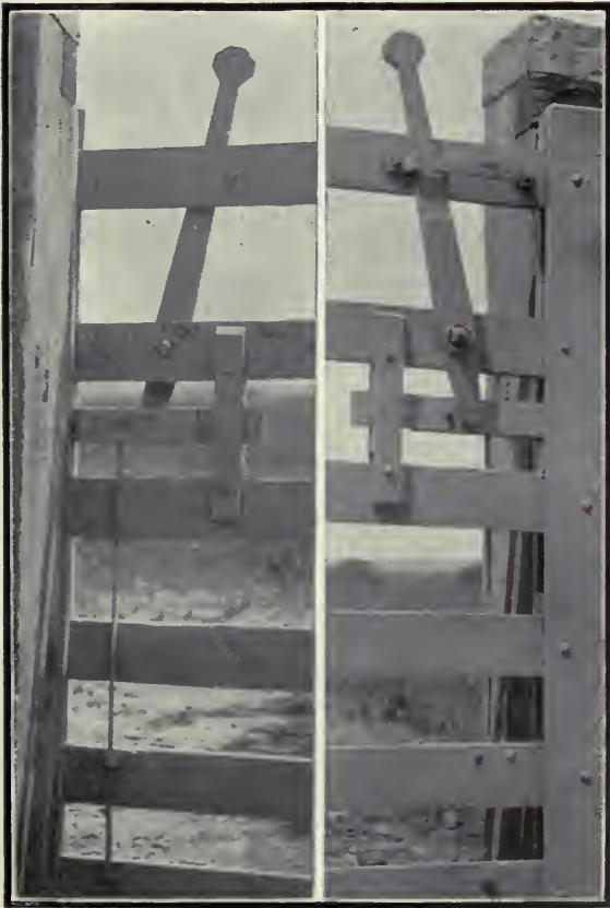
FIG. 525. FARM GATE LATCH.
