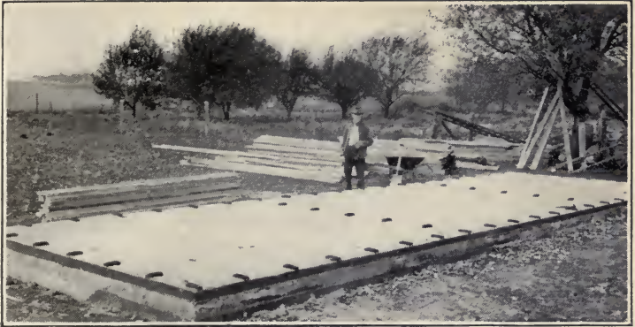
FIG. 38. — Iron Studding Sockets Set in a Concrete Crib Floor.
