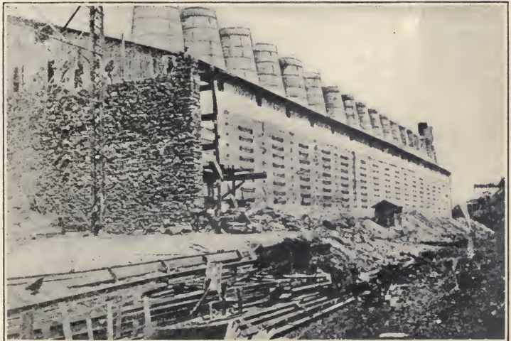
FIG. 2. — Old-fashioned Vertical Cement Kilns.
