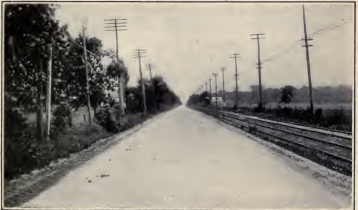
FIG. 35. — A Stretch of Concrete Road in Wayne Co., Michigan.
