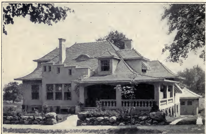
FIG. 88. — A Monolithic Concrete House, Showing Variety in Treatment and Expression.
