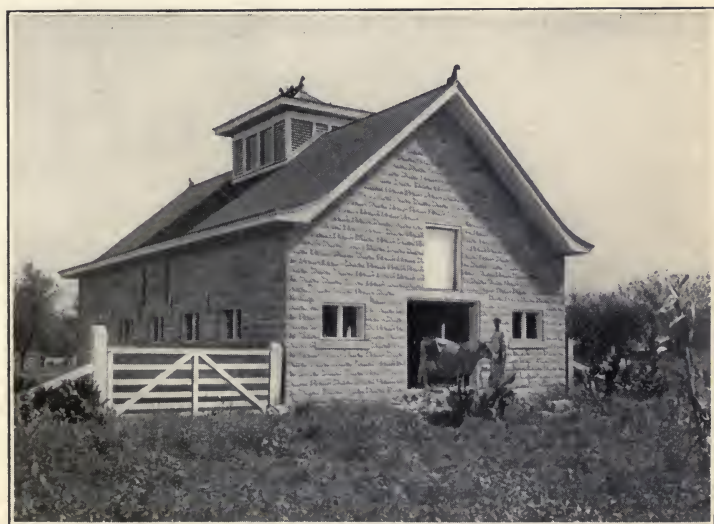
FIG. 50. — A Small Concrete Block Barn.
