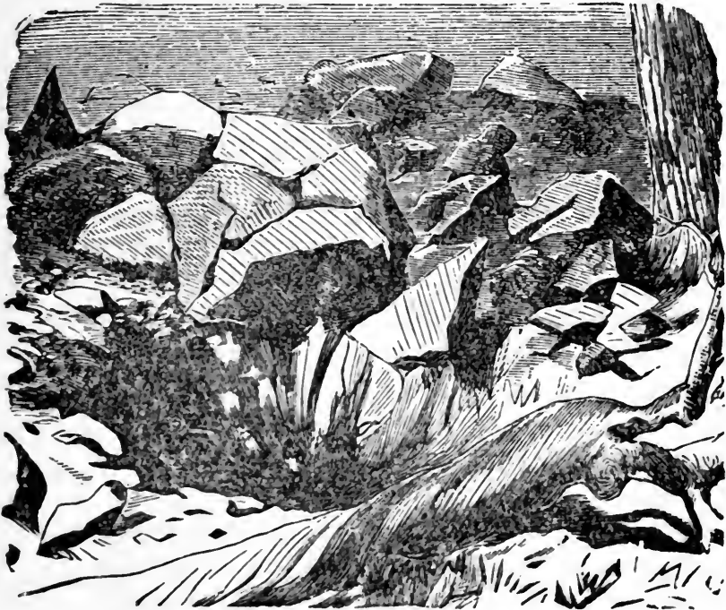
Fig. 46.—THE ROCK AFTER BLASTING.
