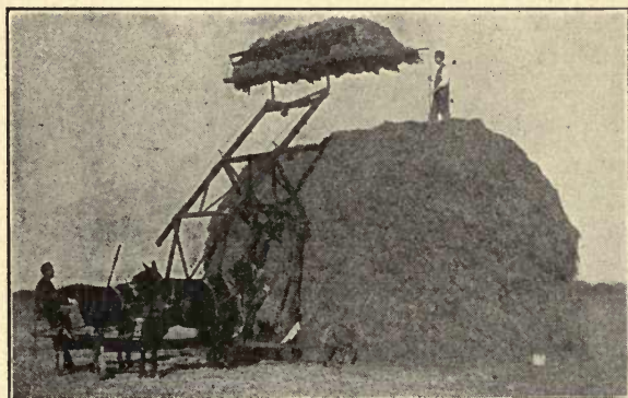
COMBINED SWEEP RAKE AND STACKER. 1
