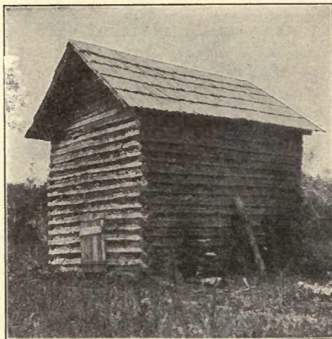
FLUE-CURING BARN, VIRGINIA.
