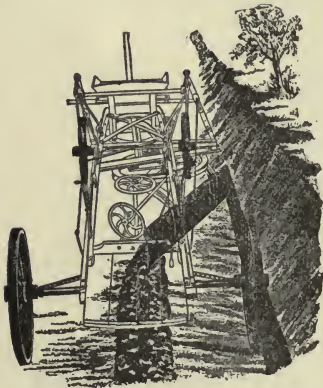
Figure 200. Reversible road machine carrying dirt from deep roadside ditch toward the center of the road.
