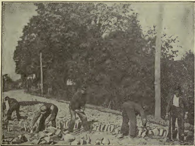
Figure 220. Laying lower course of a telford road.
