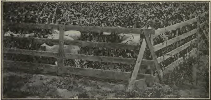
Figure 250. Light portable fence used in pasturing sheep. One piece 1 x 6 and three 1 x 4, 16 feet long, for horizontal bars; three pieces 1 x 4, 42 inches long, for up-rights; one piece 1 x 6, 42 inches long, and two 1 x 4, 60 inches long, for braces.
