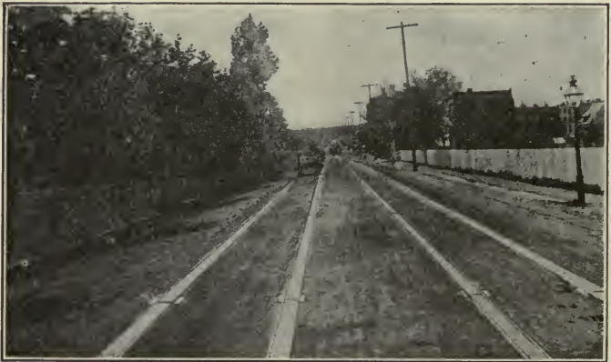
Figure 233. View of steel rails laid for wagon road.
