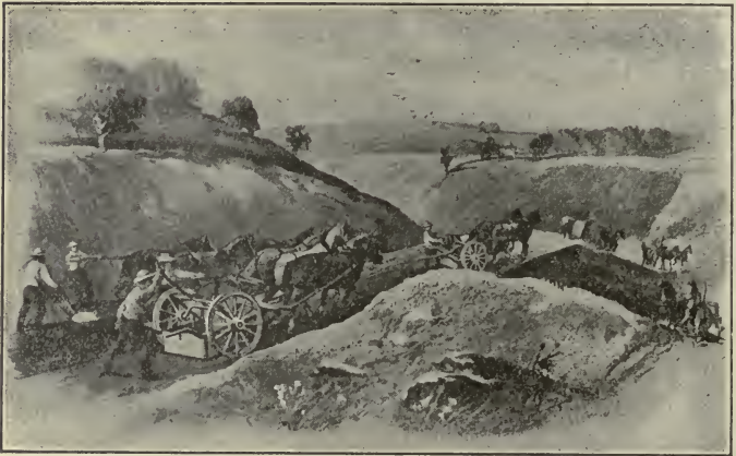
Figure 209. Wheelers, and plow, carrying earth from cut to grade.
