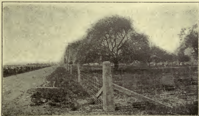
Figure 264. Well-braced cement corner post and cement line posts.
