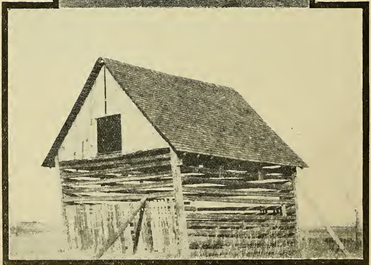
Plates 1 and 2---SMALL BARN AND POLE SHED
