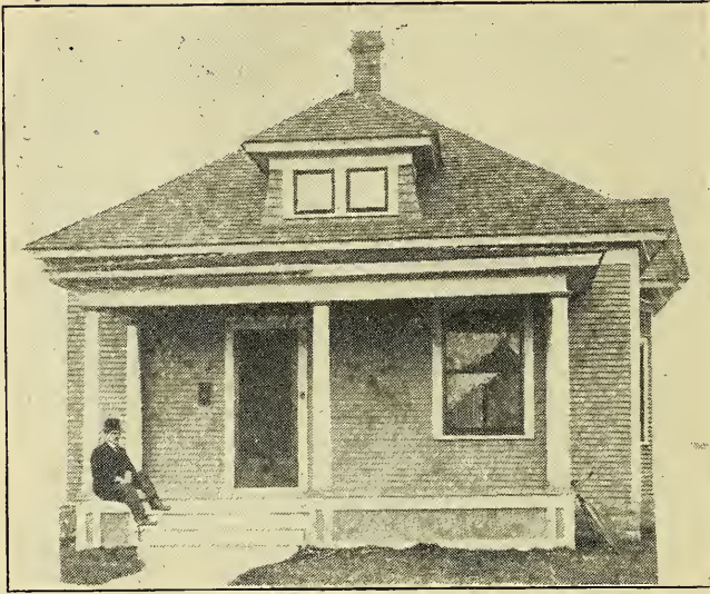
Plate 23—A NEAT FARM COTTAGE
