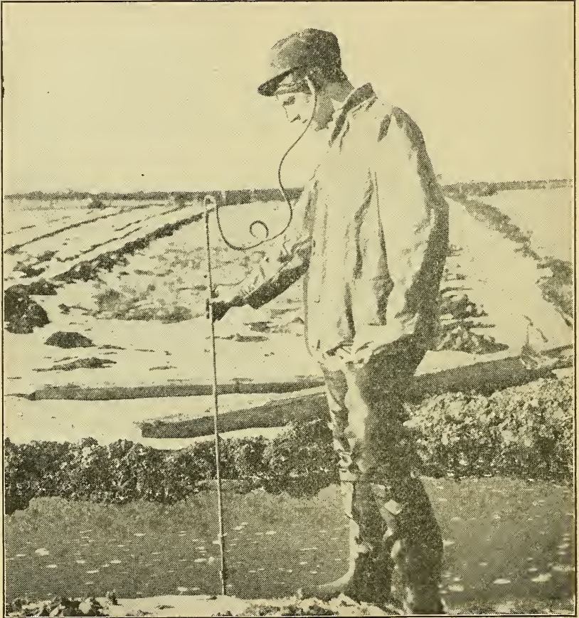
PLATE 25. The engineer in Plate 25 is measuring the flow of water in the canal by means of a current meter. There is a turbine wheel at the end of the tube which he is holding. This wheel whirls at a speed in proportion to the rate of flow of the water. As the wheel revolves it is made to give a clicking sound which is heard through the tube. The number of clicks per minute is taken and then by consulting a chart which accompanies the meter the observer is able to determine the rate of flow of the various parts of the current. The engineer in the plate is using an "Acoustic Current Meter."
