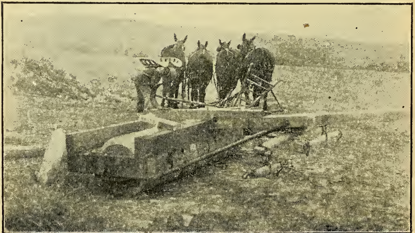
Plate 37. Very desirable land rollers are now being made by casting cement wheels in patent rims. The rims remain on the wheels and form a steel tire for them. These rollers are heavy, but due to the fact that the weight is in the wheels, they are not very hard to pull.
