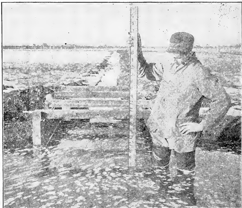
PLATE 29. Measuring the depth of the water over a weir. The rod stands upon a solid post, the top of which is exactly the same height as the crest of the weir. This measurement must be made in the nearly still water at least six feet back from the weir. (The water pitches down as it approaches the weir. There are just four-tenths of a foot of water going over their weir.)
