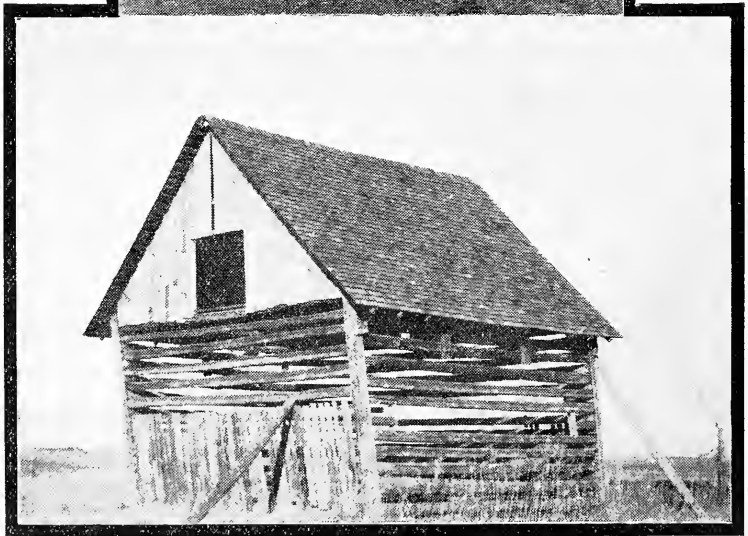
Plates 1 and 2---SMALL BARN AND POLE SHED
