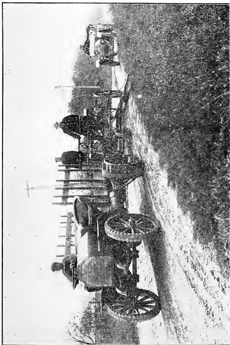
Plate 24. A patent road drag or "surfacer" dragging a road at the proper time to give a smooth, hard finish to the surface. Such a machine coupled to a strong tractor makes a very good combination as the work of dragging can be done with great rapidity at exactly the right time.
