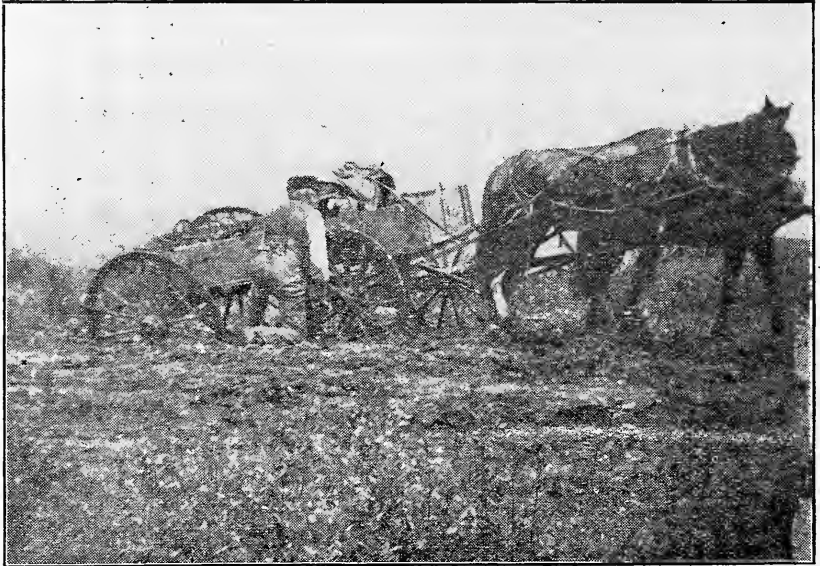
Plate 6. A little scientific road drainage would have prevented this condition of the road shown in the plate.
