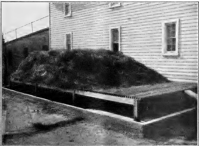
FIG. 14.—A maggot trap for house-fly control. View of the maggot trap, showing the concrete basin containing water in which larvæ are drowned, and the wooden platform on which manure is heaped. (Hutchison.)
