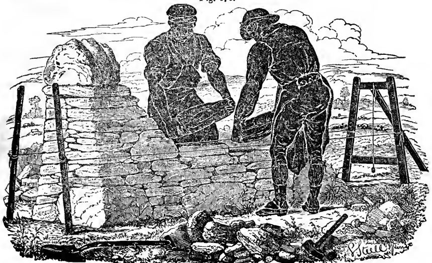
THE BUILDING A DRY-STONE DYKE.
