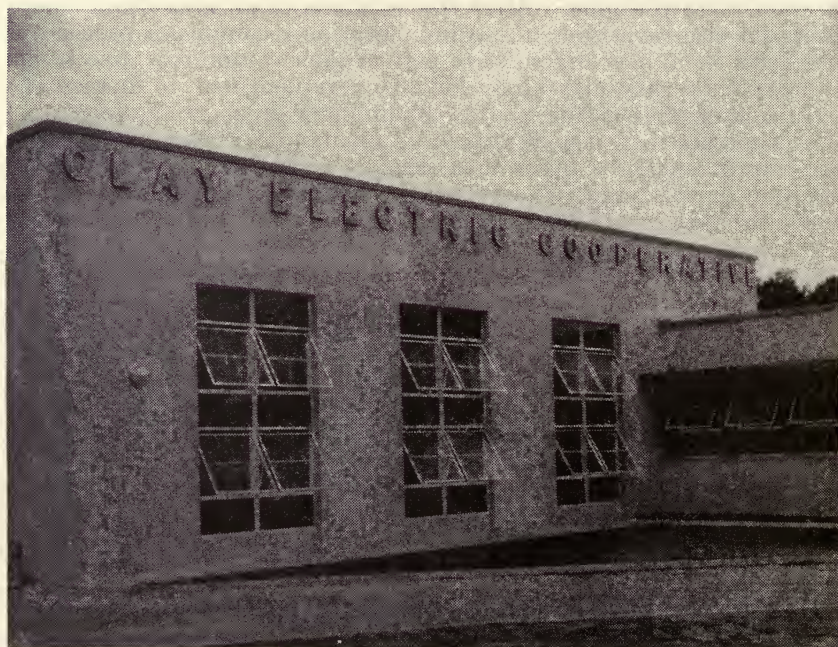
Figure 2.—Such a generating plant as this may be built by a cooperative with money borrowed from the Rural Electrification Administration when electric power from existing sources is not available or cannot be obtained under satisfactory conditions.
