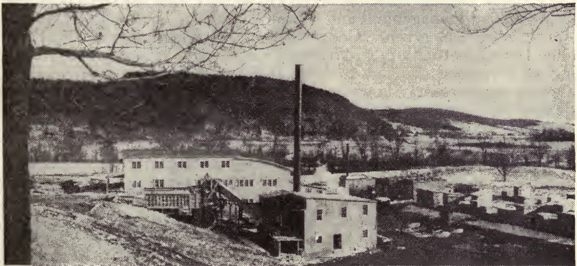
Figure 4.—Plant of the Otsego Forest Products Cooperative Association, Cooperstown, N. Y. This is a pioneer effort still in the experimental stage, designed to prepare hard-wood timber suitable for the general market for sale at full value and to saw and plane local hemlock and pine for use on farms and in the community. Fuel wood, sawdust, and other byproducts are also available to farmers.
