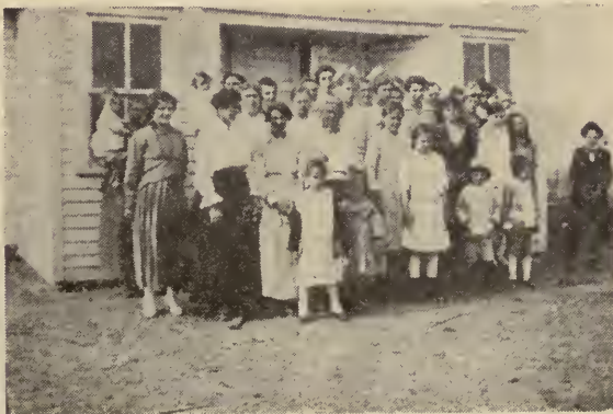
TROY POND SCHOOL, KILBOURNE TOWNSHIP
