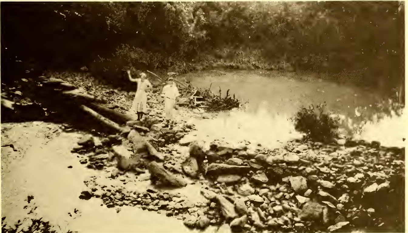
Fuller Rock Bridge, 1933, Uwharrie River. Built by Allen Fuller.
