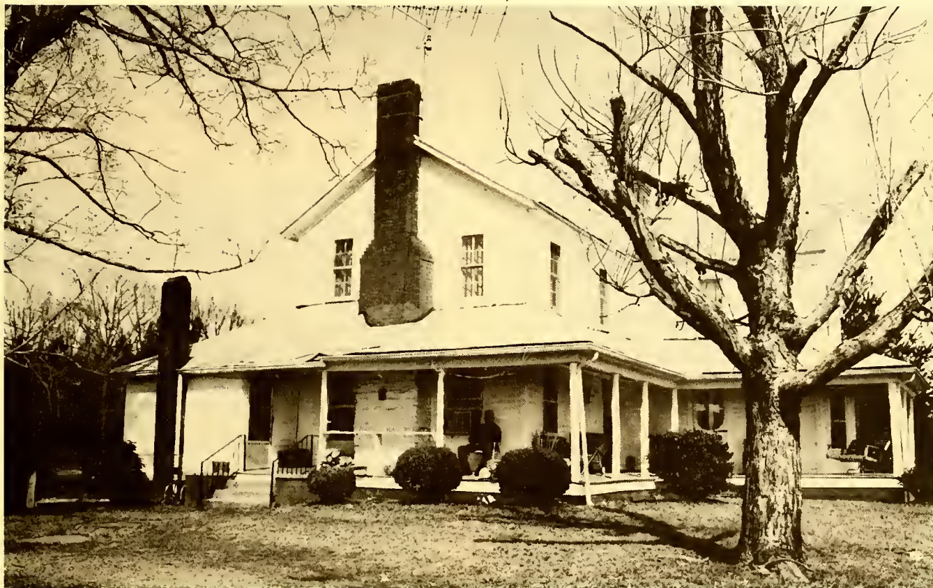
The Marsh Dorsett house originally. Began as a four-room dwelling and remodeled in 1920 by the present owner, Carson Cranford.
