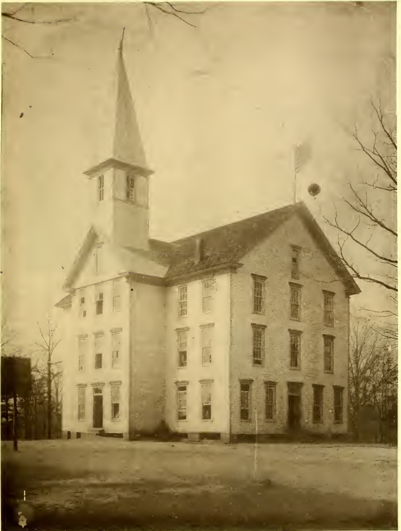
The Farmer High School building that burned in 1923. Built in 1893, it served as the "Farmer Institute" until 1907 when it became a public school. An academy building preceded the above structure.
