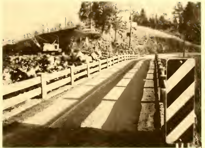
The bridge at Parker's Mill. At left, excavation for a new dam to store water for the City of Asheboro.
