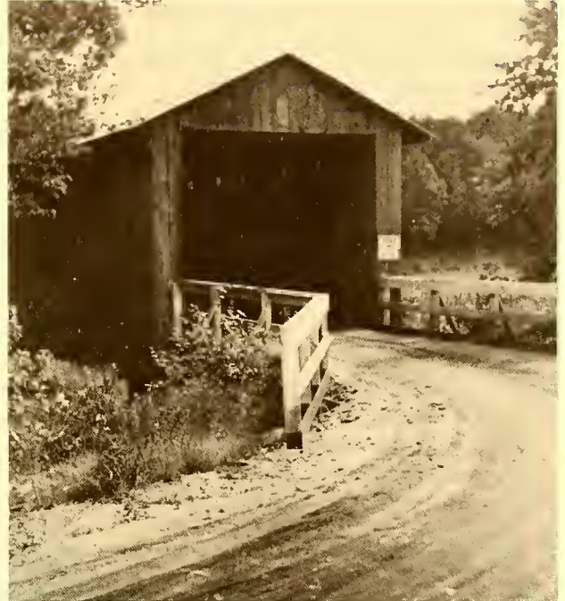
Lassiter’s Mill Bridge
