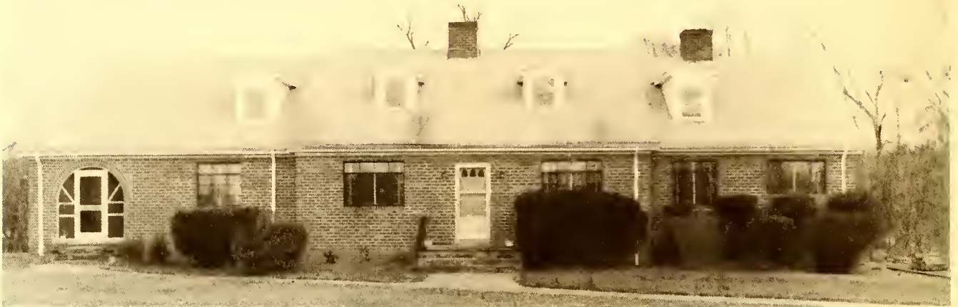
“Dump” Lassiter’s home. Bricks made of clay dug from the farm. Charles Lassiter, a son, drew the plans and supervised construction.
