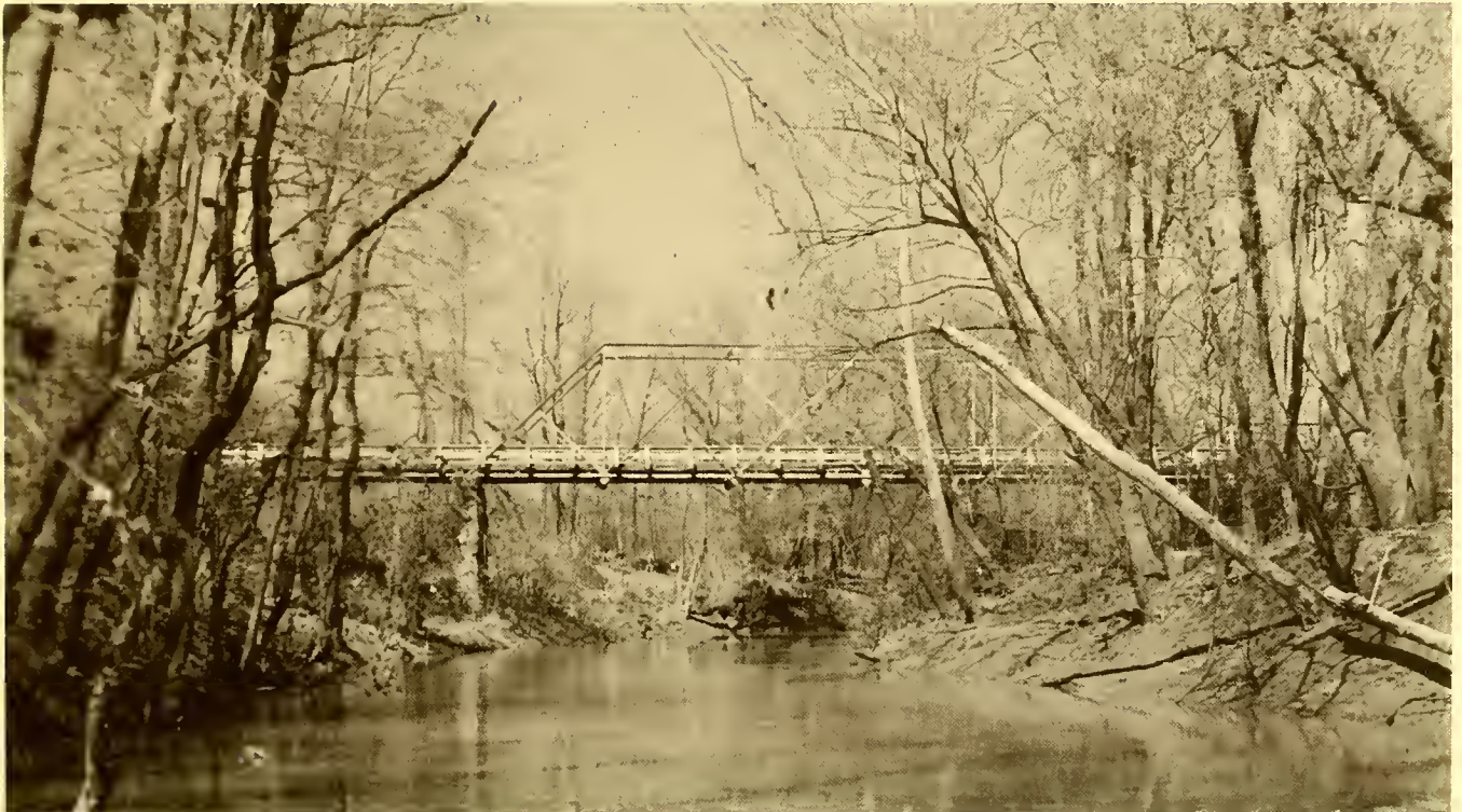
Dunbar Bridge over the Uwharrie River between Mechanic and Farmer, N.C.
