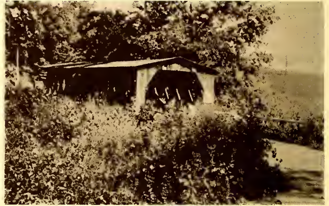
Tom's Creek Bridge near Farmer
