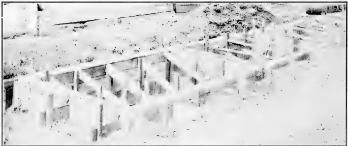
FIG. 12.—Showing the method of constructing a concrete hotbed. Note the framework which is necessary.
