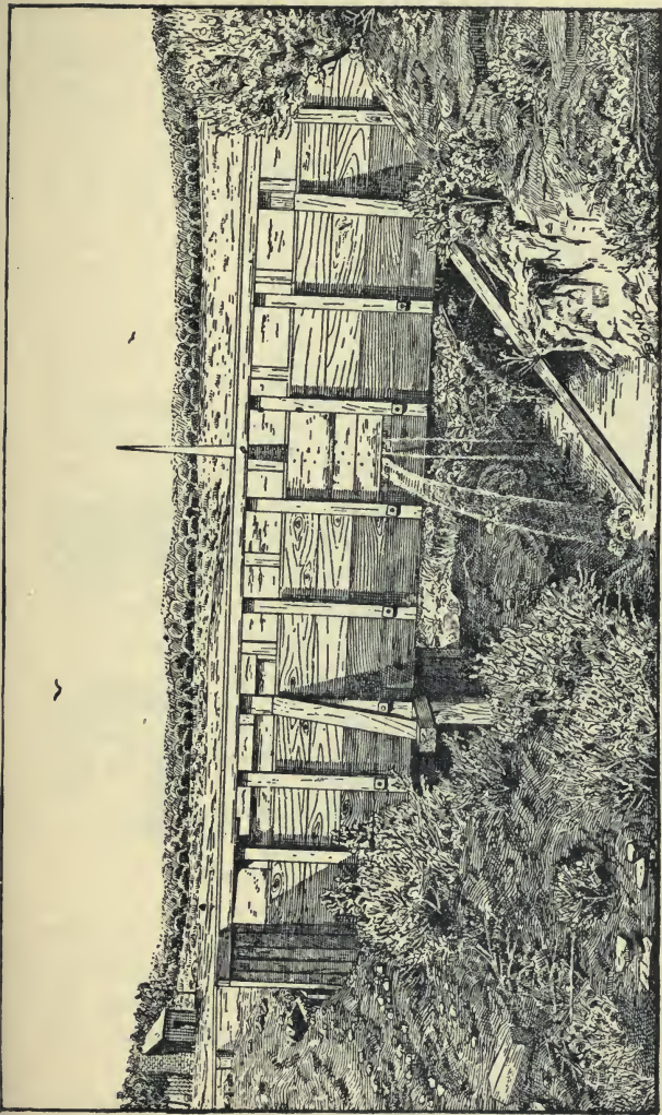
FIG. 29—BOX FLUME WITH WASTE GATE.
