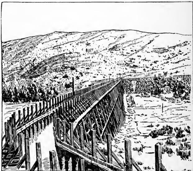
FIG. 30—FLUME ACROSS A VALLEY.
