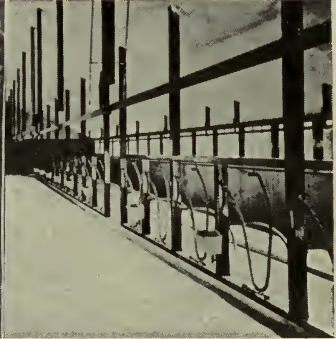
FIG. 213 A.—Bad construction. Difficult to keep clean. (Animal Industry.) FIG. 213 B.—Good construction. Smooth floor, walls, and ceiling, plenty of light, easy to keep clean. (Animal Industry.)
