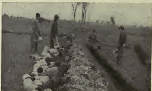
FIG. 38.—Ready to lay the six-inch drain tiles.
