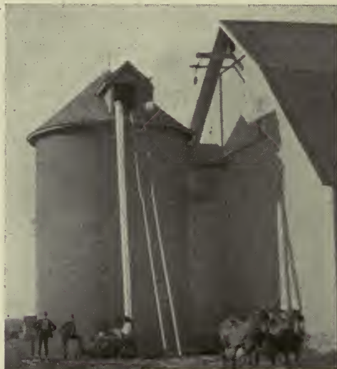
FIG. 209.—A modern brick silo near end of dairy barn. The cutter and pipe through which cut corn is blown are in place to begin filling silo.
