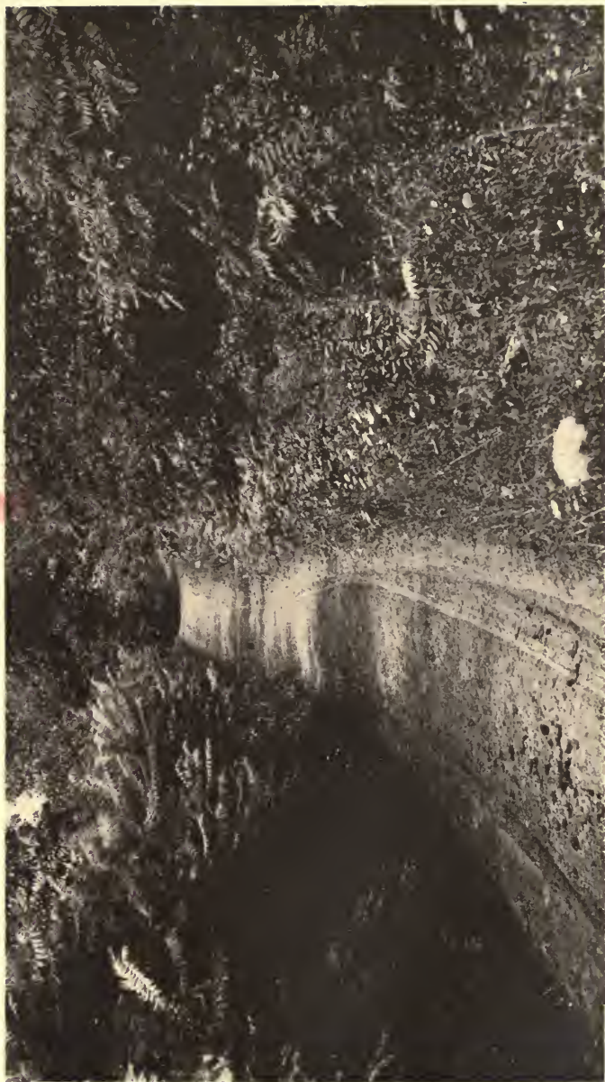
43. A STEEP HILL ON THE TOP OF WHICH SEVERAL FINE FARMS ARE LOCATED It is a mile and a quarter long, with a grade of 3 inches per foot in the steepest place, 20 feet rise in 100 being frequent
