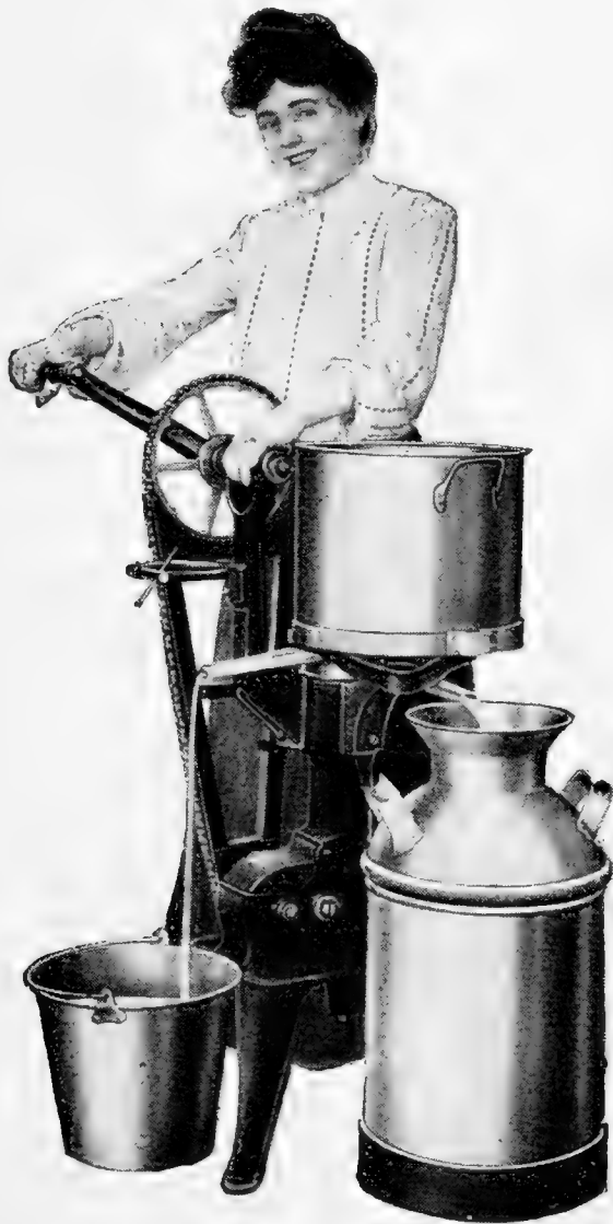
SEPARATING BY HAND WITH CHAIN DRIVE CREAM HARVESTER "DAIRYMAID."
