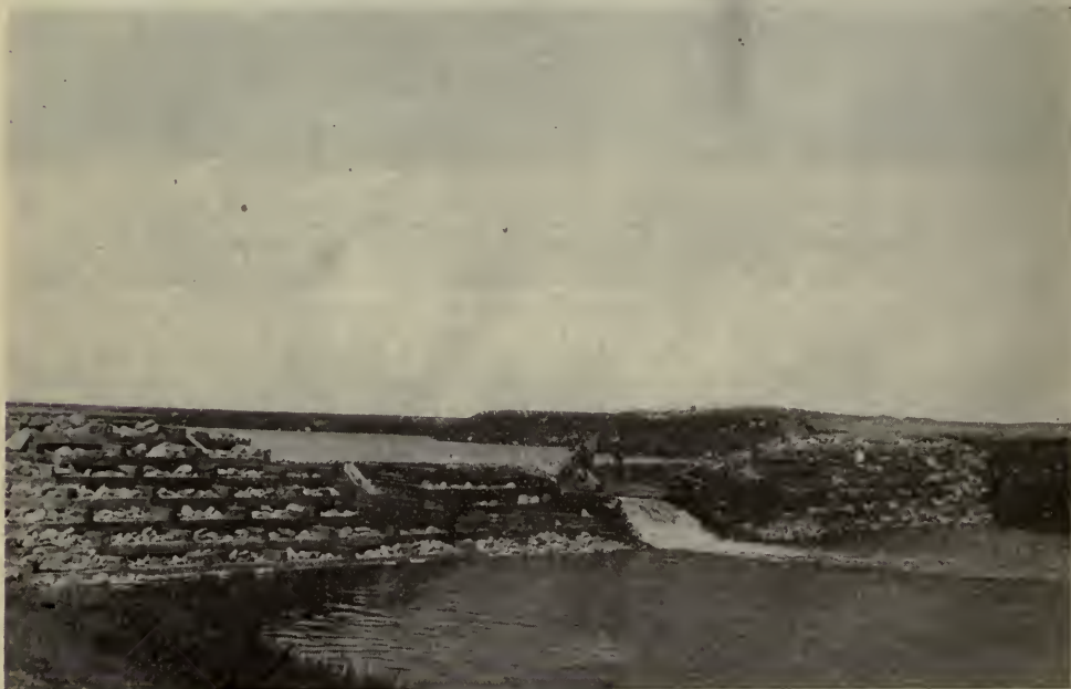
General view of rock-filled crib dam. This is a good type where timber and rock are plentiful. Photo shows the type of construction with square timber. Round timber notched out at the joints makes just as good a dam. This dam has a wood spillway, but the whole top can be made level and to act as a spillway. The water side of the dam has to be faced with planks or banked up with earth to stop leakage.
