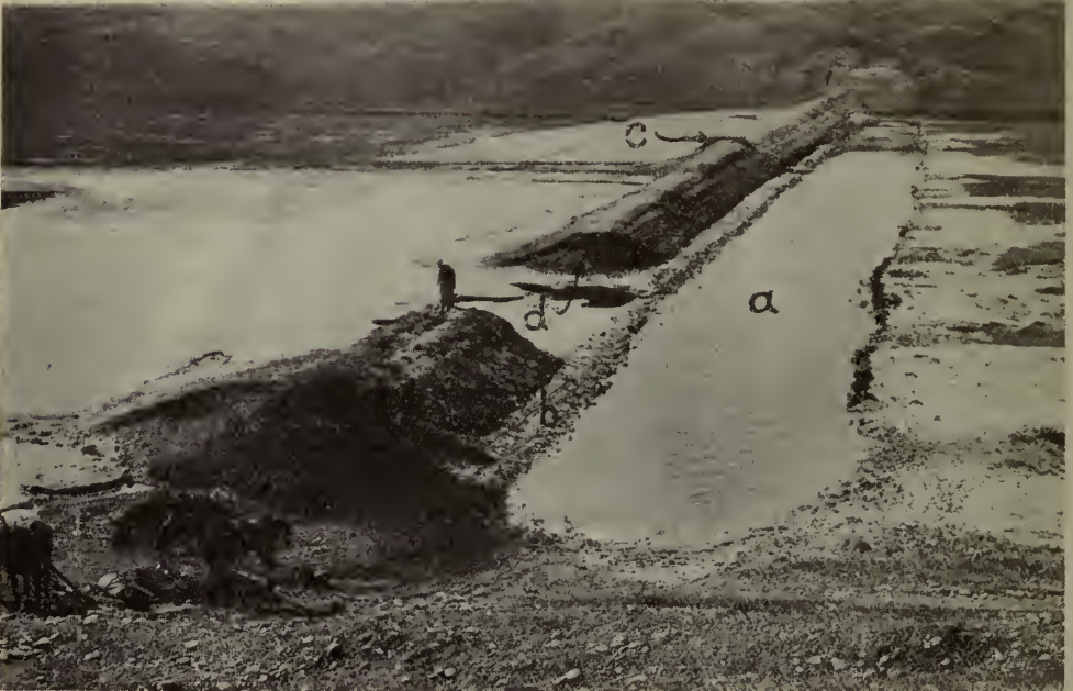
General view of an earth dam built across a wide flat coulee. (a) shows the idea of making a combined dugout and reservoir by building the dam entirely from excavation from one borrow pit in the bottom of the reservoir. (b) shows the "berm" between the toe of the dam and the borrow pit. This is too narrow and the dam would be stronger if the excavation was a little further away; this is a common fault and should be guarded against. (c) Wood spillway through centre of dam. (d) The face of this break gives a good idea of what the cross-section of this dam is, showing the top and bottom widths and the side slopes.
