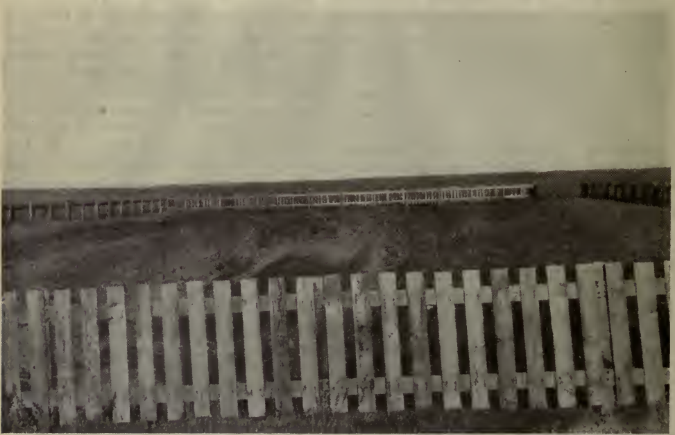
This shows the type of dugout which has been used successfully in Saskatchewan. The fence is built not only because it keeps out stock but also because it catches a lot of snow during the winter which melts and helps to fill up the reservoir in the spring. This dugout was started without first testing the kind of soil, and the bottom is in such sandy soil that the water leaks out.
