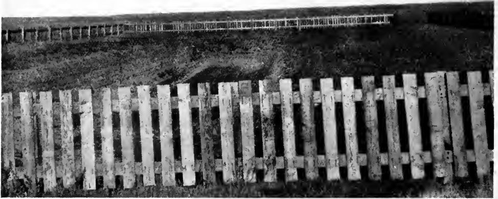
This shows the type of dugout which has been used successfully in Saskatchewan. The fence is built not only because it keeps out stock but also because it catches a lot of snow during the winter which melts and helps to fill up the reservoir in the spring. This dugout was started without first testing the kind of soil, and the bottom is in such sandy soil that the water leaks out.
