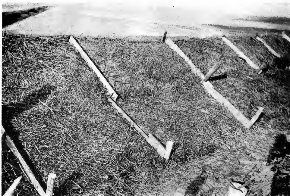
Close up view of an earth dam protected on the wet side with riprap made of straw held down with chicken wire and wood posts driven into the earth. Old boards have been nailed between the wood posts instead of using wire.
