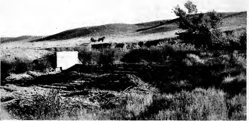
General view from down-stream side of rock and brush dam built across a creek. The dam is built up of alternate layers of brush and rock. The rock works down into the brush and so does not show up much in the photo. Note that the dam is started on a broad base and then gets narrower towards the top. This kind of dam is leaky until it gets filled up in front with mud and silt. This dam has flash boards placed on top of the crest but these are not necessary for the ordinary farmer's reservoir. This kind of dam is liable to be damaged if heavy ice comes down in the floods and is not as good as the wood and rock type of dam.
