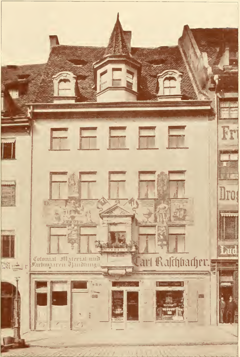
THE "BEHAIM" HOUSE AT NÜRNBERG.
