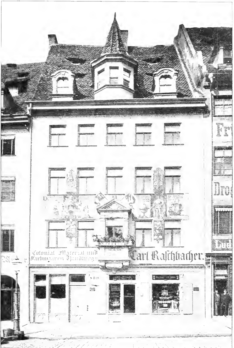
THE "BEHAIM" HOUSE AT NÜRNBERG.
