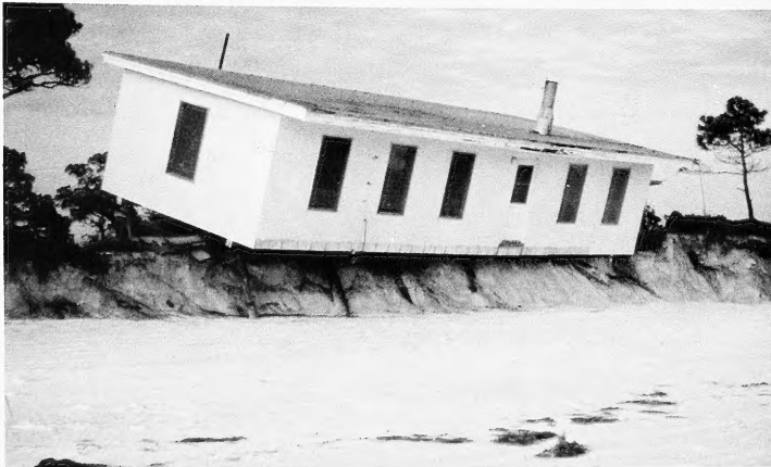
Figure 1. Storm damage caused by erosion of the dune
