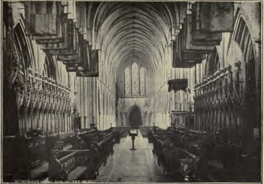
INTERIOR VIEW OF ST. PATRICK'S.
