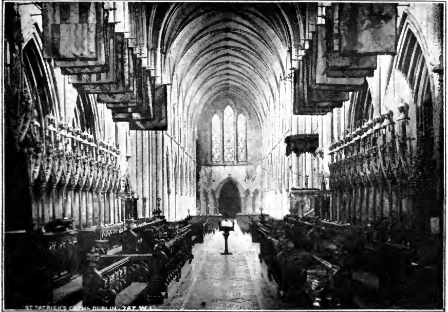
INTERIOR VIEW OF ST. PATRICK'S.
