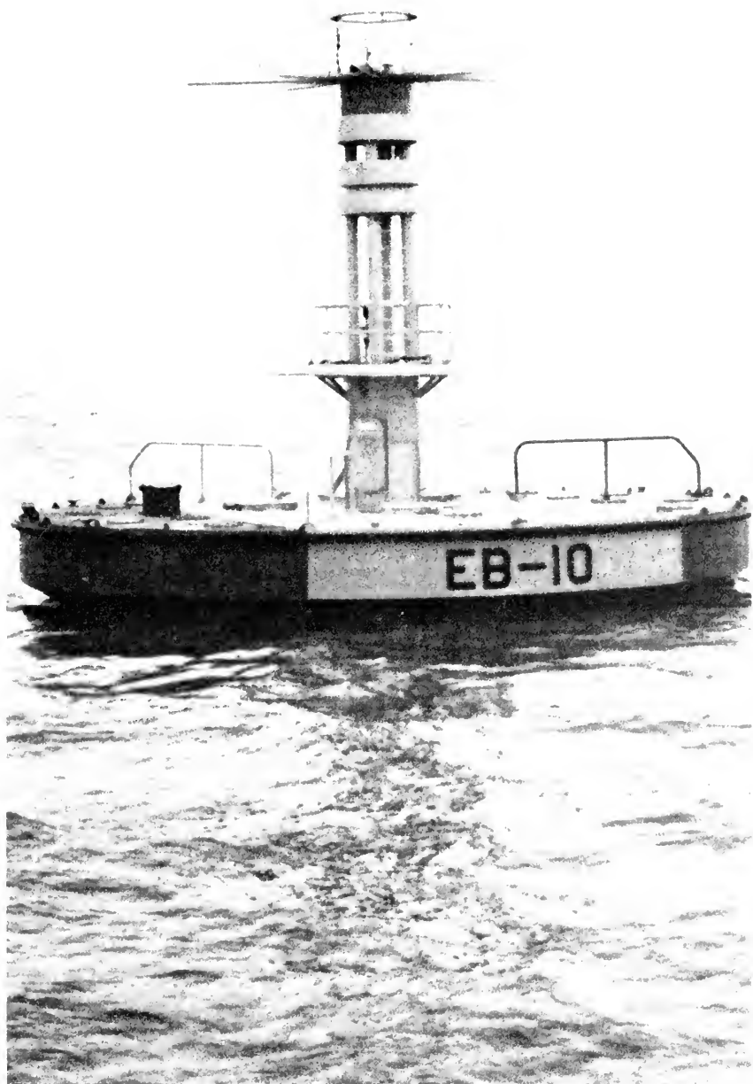
The first of a series of six EEP buoys being readied for stationing in the summer of 1972. These 100-ton platforms, designed to withstand 150-knot winds, 60-foot waves and 10-knot currents, will be anchored in almost two miles of water 225 miles from Gulfport, Mississippi and can carry more than 100 sensors to measure and report oceanic and atmospheric conditions.
